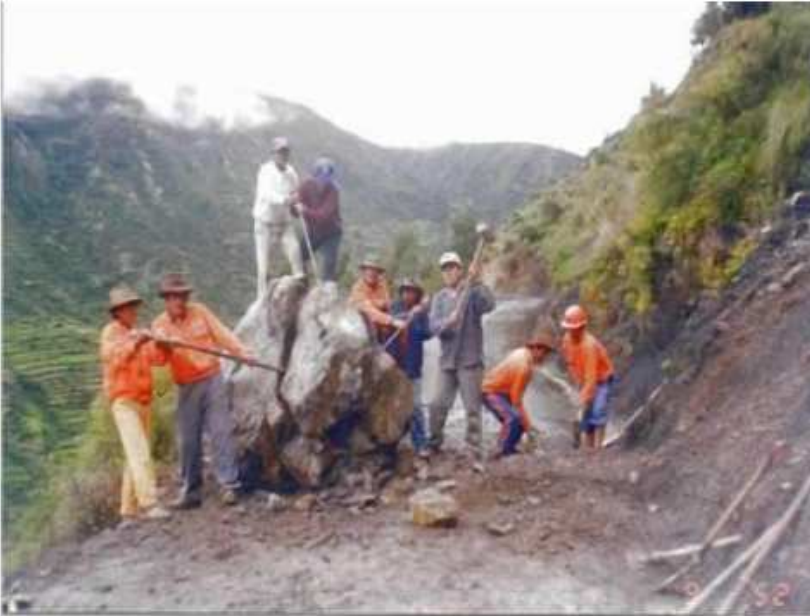
Figure 3: Treated Roads – Examples of maintenance work
